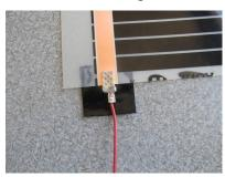
4. No matter which way you use the mounting spot is insulated carefully with safety tape from both sides – ph4 and ph5
