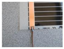
2. This is mounting of the cold ends by soldering (the better way) – ph2.
