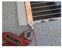
3. This is mounting of the cold ends using clips and plyers – ph3.
